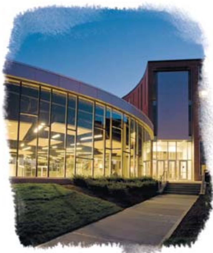
LEED Platinum Certified Student Innovation Center
